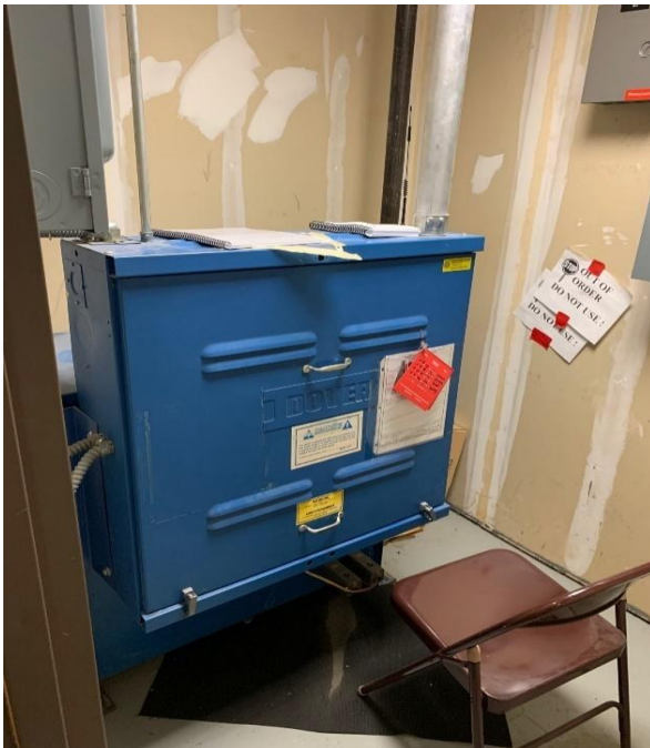
Photo Description: Elevator.
